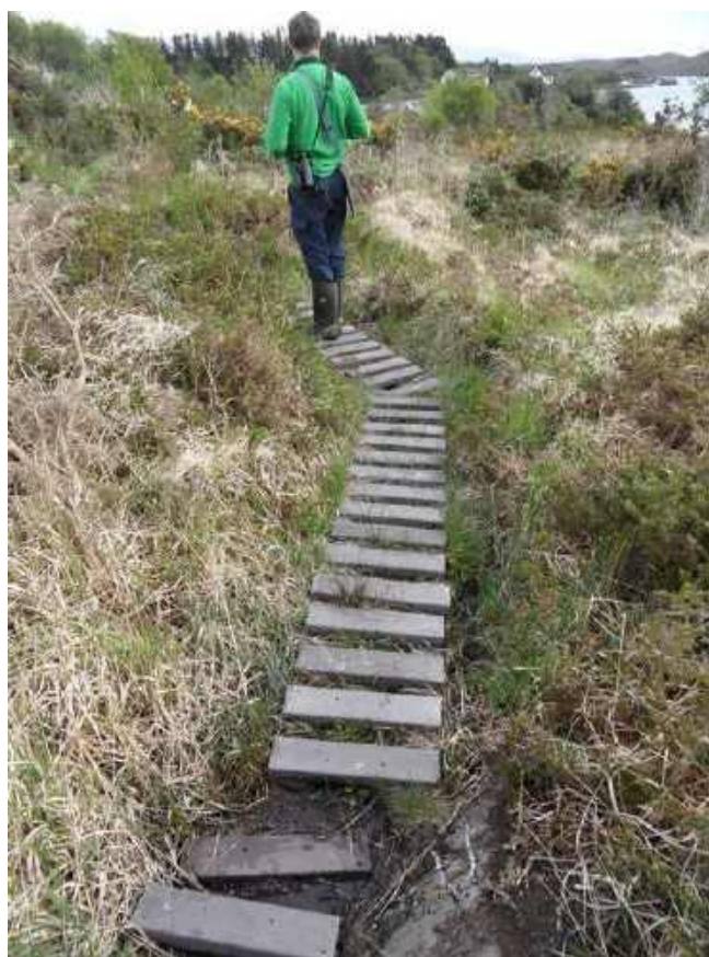
Plate C6: Steps on the southern edge of the peninsula in Area C. The path along the route from the quay to the Sneem Hotel is in poor condition in parts. Upgrading of the path and steps is recommended.
