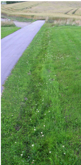
Roadside swale in north Cork, with earthen check-dams and pocket pools planted by volunteers as part of local community scheme.
