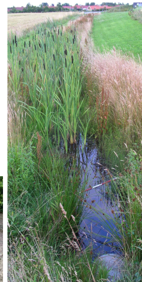
Two swale examples from a stormwater drainage system in Denmark taking village urban runoff. Dry grassed swale (L) and wetland planted swale (R) both filter water en route to a stormwater wetland lower in the catchment.
